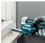
Removal of window frame
